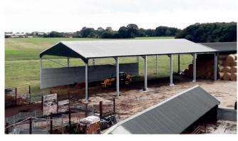
cement roof and concrete panels for one wall at the back. Footings went in during March and all was looking good for completion before harvest time. This would be ideal as we could then put straw produced from this year's harvest straight in. It
